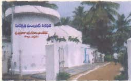
Water purification plant at Kovvada-Annavaram
